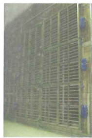
4 Hrs FRP Damper with Actuators (Electrical Drive)
