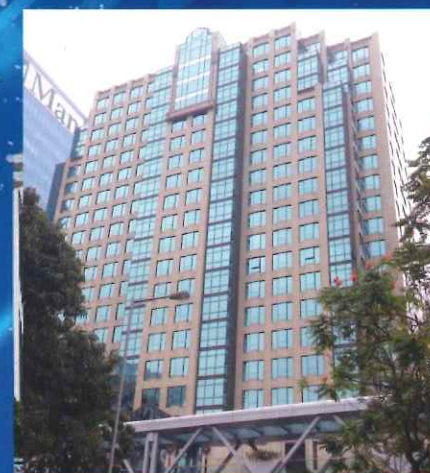
Electrical & Mechanical Package and Revitalisation of Industrial Building in Kwun Tong Lu Plaza (2016 - 2017)
