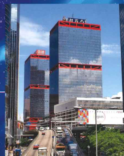
MVAC Installation Works for the Building Renovation and Improvement Works in Shun Tak Center (2016 - 2018)
