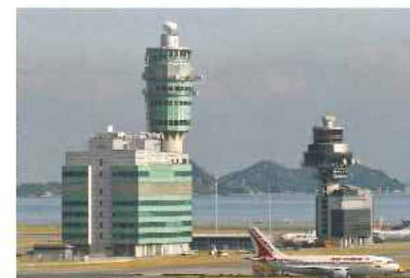
Air Traffic Control Complex and Tower - Chek Lap Kok Airport
